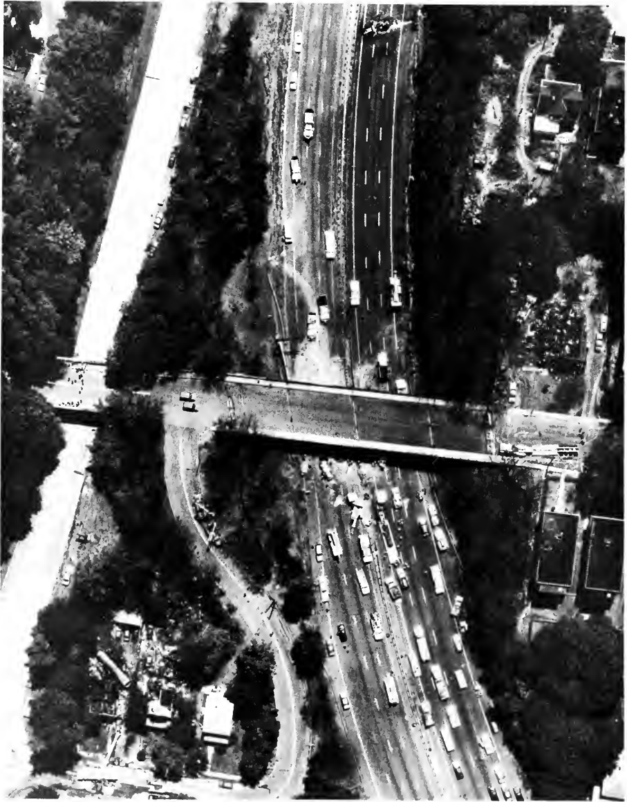
Figure 2. -- Aerial view of accident site (Photo by Chas. H. Sells, Inc.)
